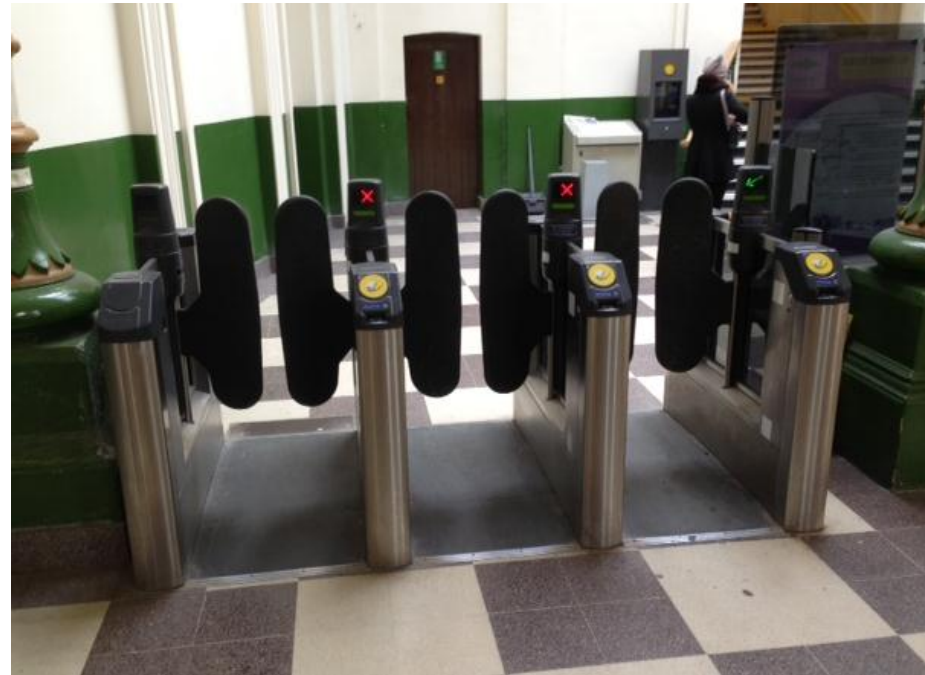
FIGURE 2.2 UTS GATES AT BATTERSEA PARK STATION
